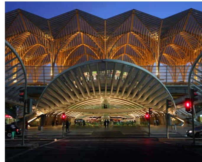
Túnel Metro de Lisboa / Subway Tunnel in Lisbon
